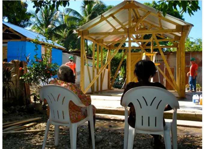
Transitional shelter being built, while people look on.
